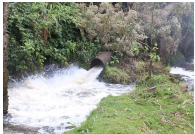
Figure 50: Incomplete Penstock at the Ina-Njugu Micro-Hydro Power Project
