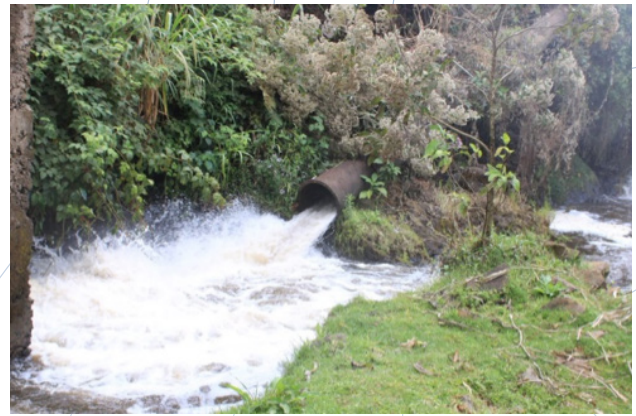
Figure 24: Site Visit to the Ina-Njugu Micro-Hydro Power Project - Uncompleted Penstock (Day 3)
