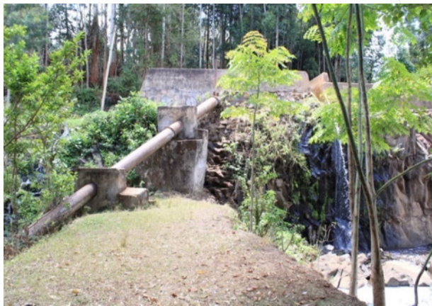
Figure 47: Penstock at the Kianguruwe Mini-Hydro Power Project
